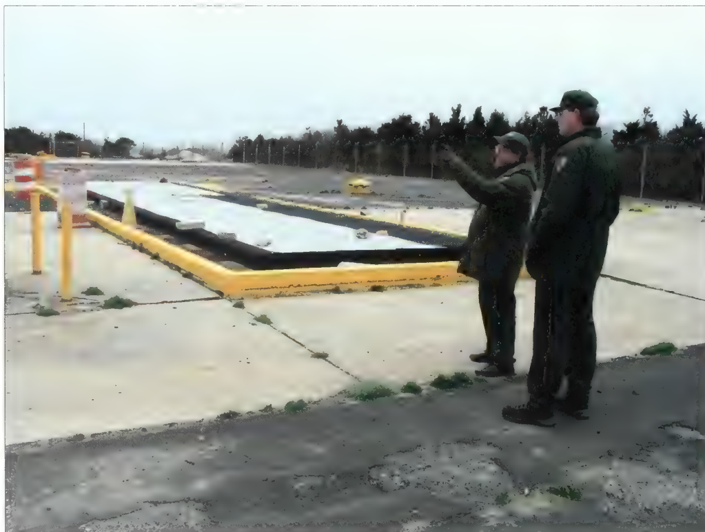
Figure 3.64. View looking west at elevator to missile magazine (425), NIKÉ launch site. The northern section of the launch site contains the underground missile magazines and concrete pads for launching racks. The concrete pads are oriented north to south for firing missiles to the east (Olmsted Center, April 2008).
